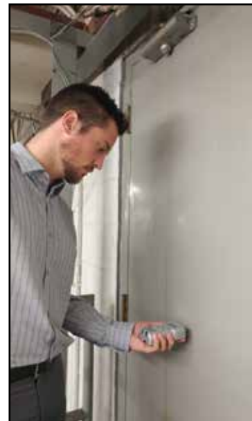
Checking door force to access pressurized stairwell.
